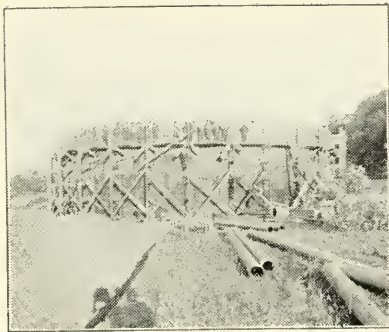
BUILDING AN OIL TANK.
